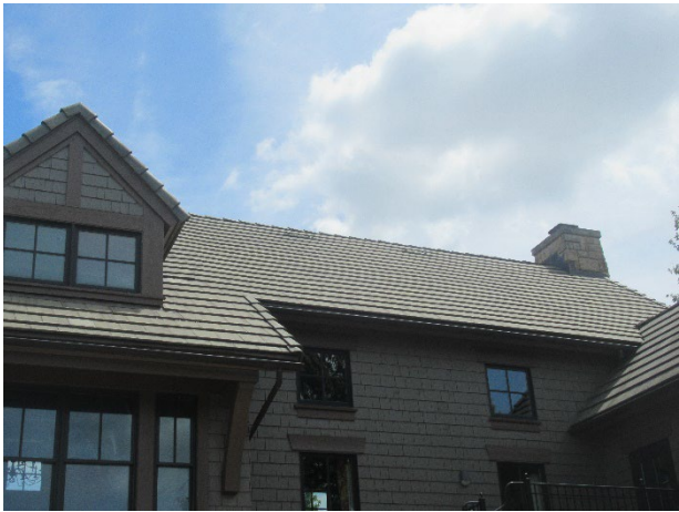
Tile roof overview
