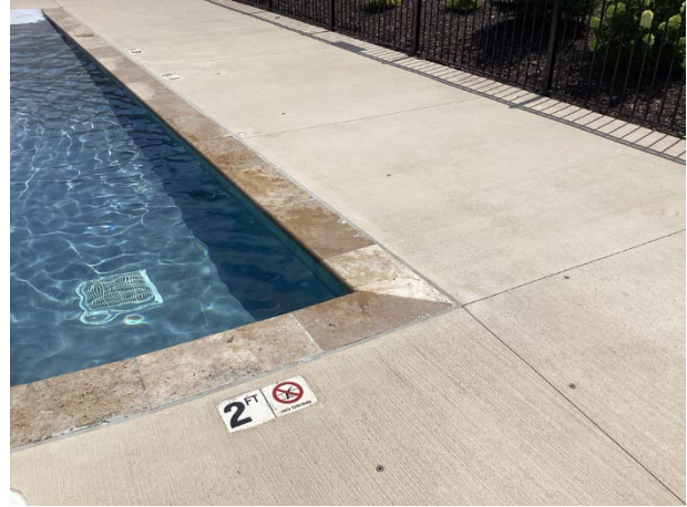
Concrete pool deck and coping
