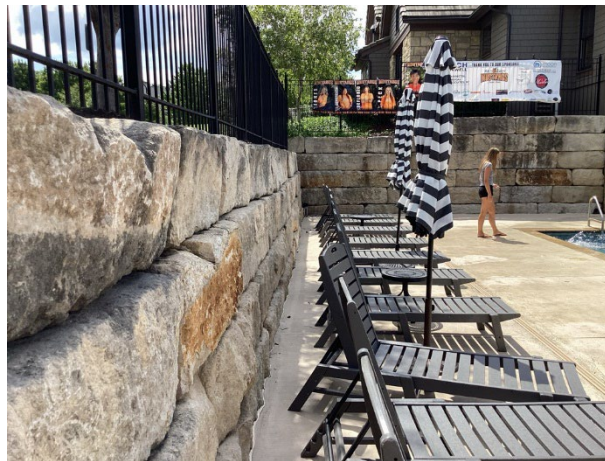
Stone retaining wall
