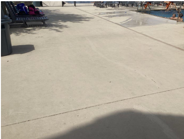
Concrete pool deck overview
