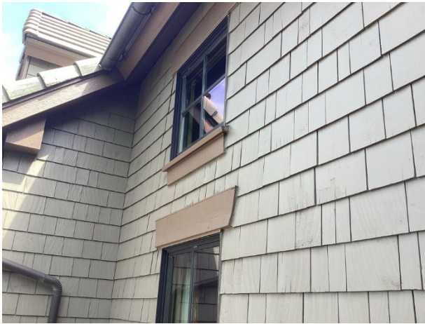
Siding and trim overview
