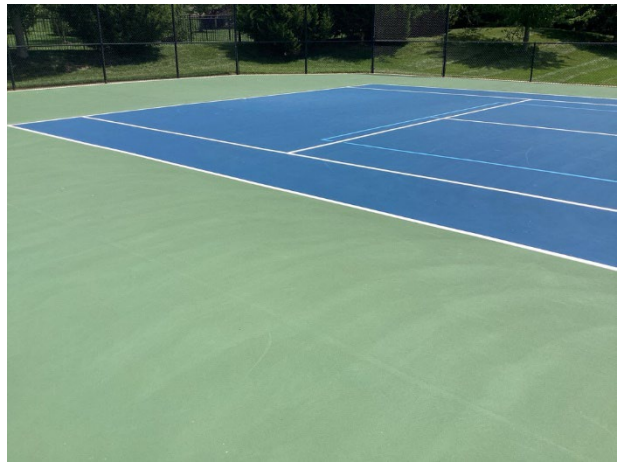
Tennis court overview
