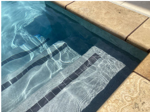
Lap pool plaster finish with tile perimeter
