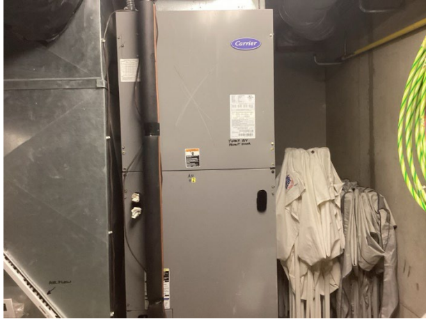
Split system air handling unit
