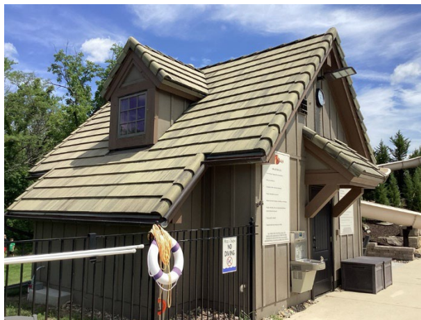
Pool pump house
