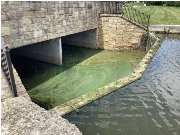
Pond spillway towards other pond
