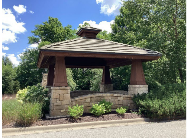
Entrance monument structure with concrete tile roof
