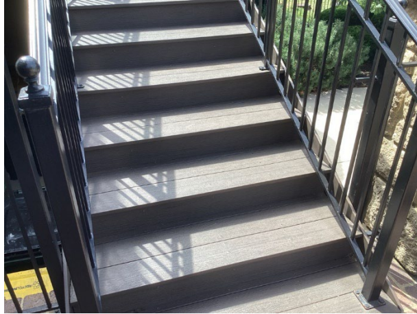
Composite treads at wood frame staircase
