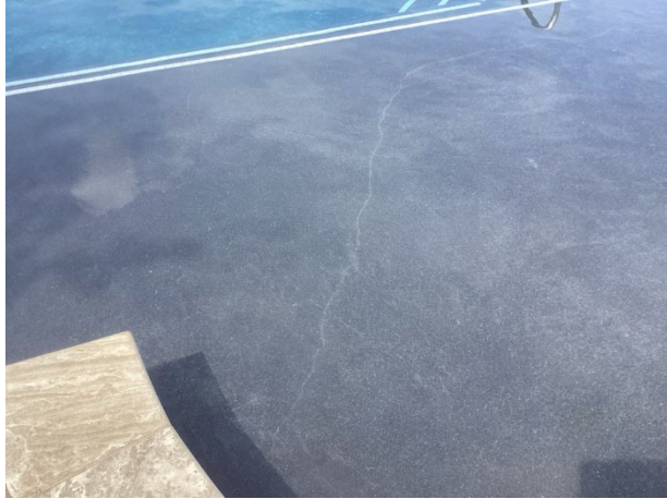
Plaster cracks
