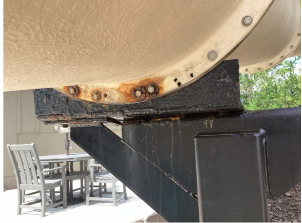
Rusted fasteners
