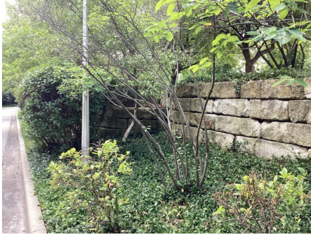
Stone retaining wall near King St entrance
