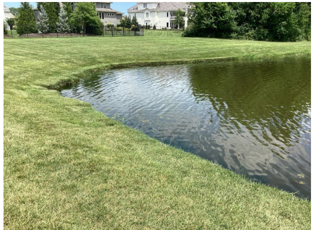
Minor shoreline erosion
