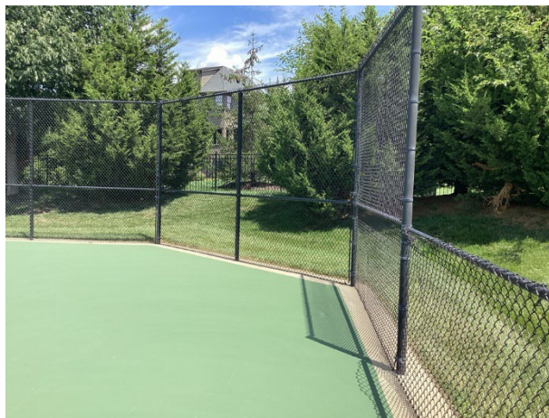
Chain link fence
