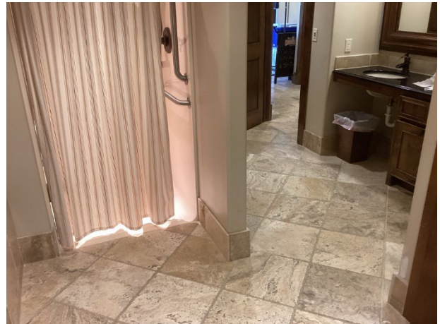
Shower and finishes at lower level
