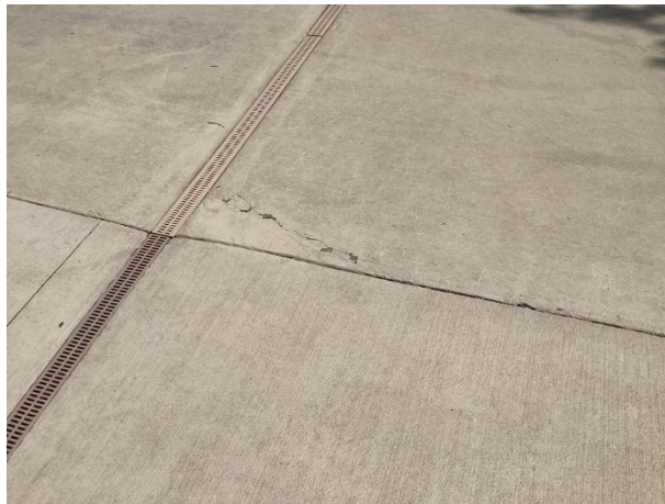
Concrete cracks
