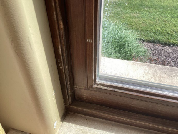
Wood deterioration
