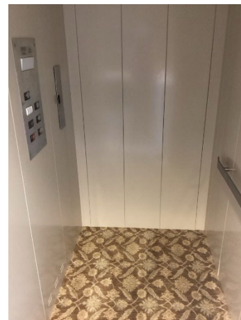
Elevator cab interior
