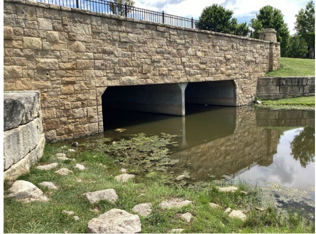
Culvert structure, note long-lived
