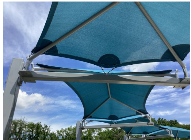
Shade structure overview
