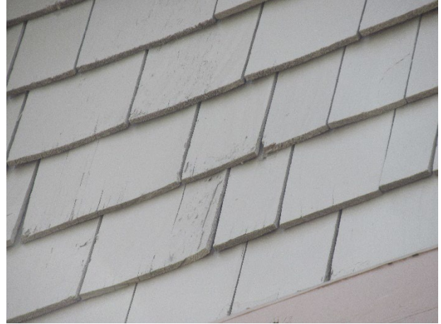
Siding deterioration
