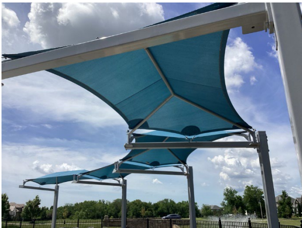
Shade structure overview
