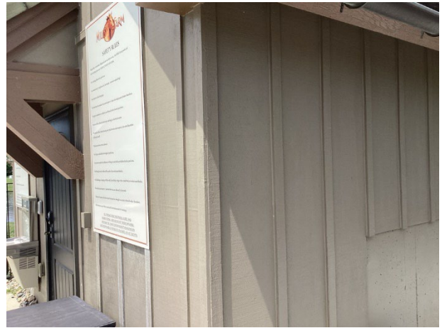
Composite hardboard siding at pump house
