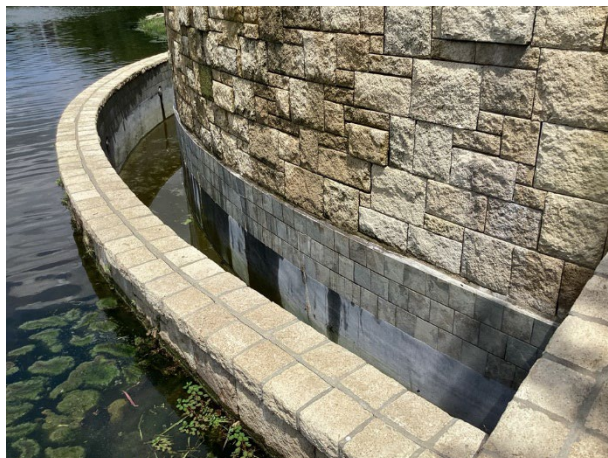
Infinity pool structure
