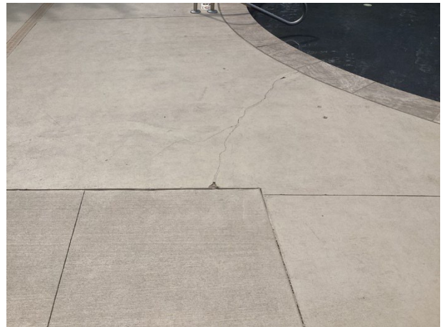
Concrete cracks
