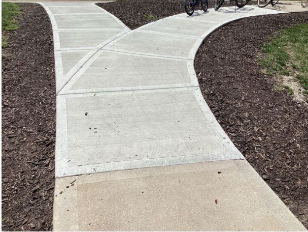
Sidewalk partial replacement by pool
