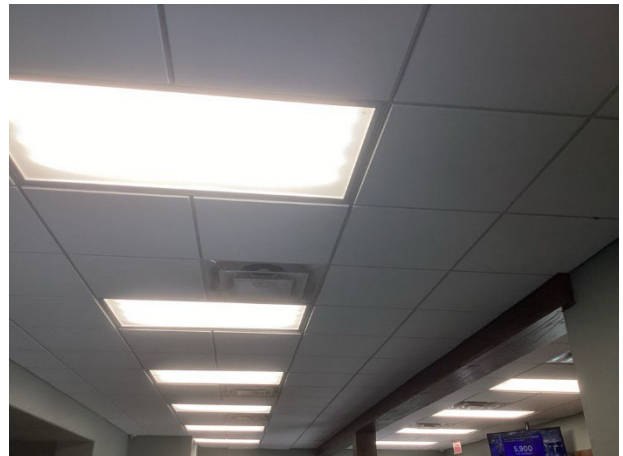
Acoustical ceiling tiles and lighting
