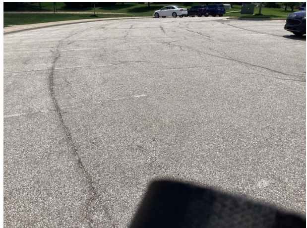
Pavement cracks
