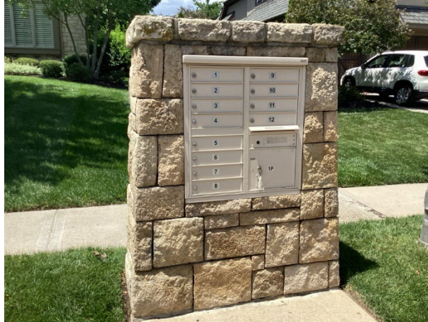
Mailbox station with stone masonry exterior
